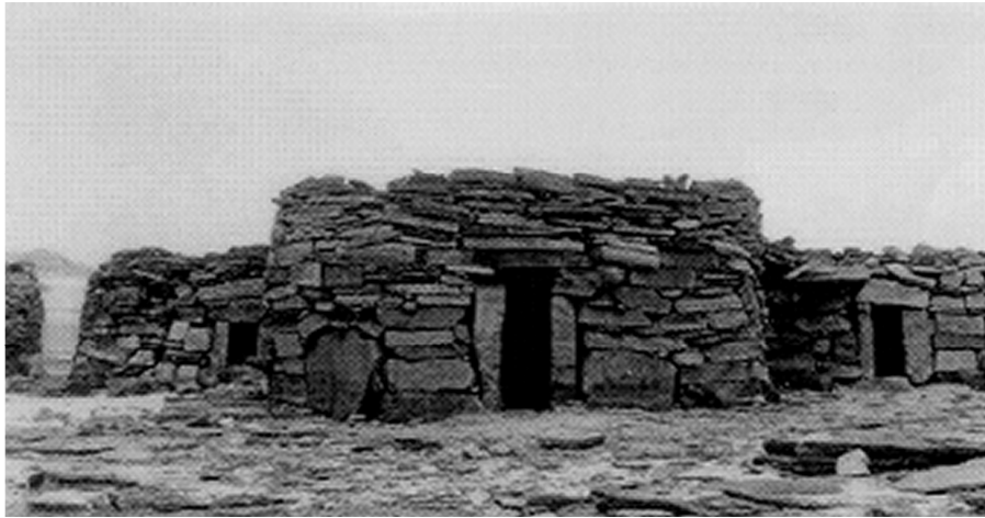
Fig. 2. Nawamis structures (photo: I. Hershkovitz)
