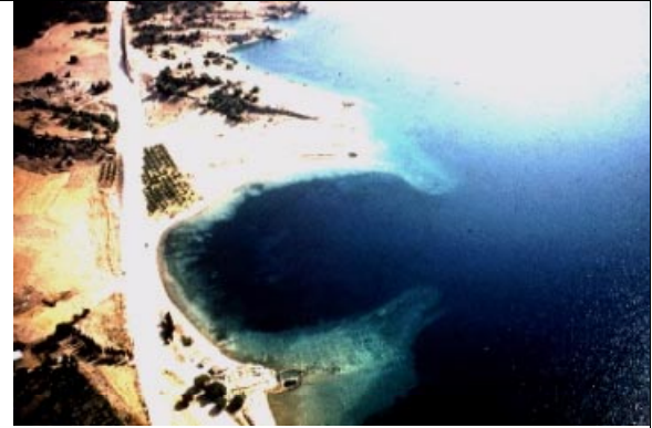
Figure 13: Submerged harbor works.
